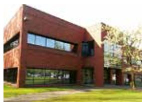
FLIR Systems, Portland
